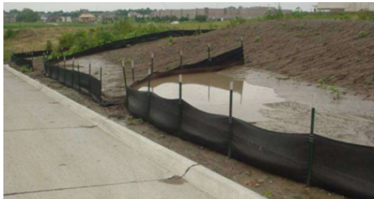
Figure 6-3. Typical Example of a Silt Trap fence
